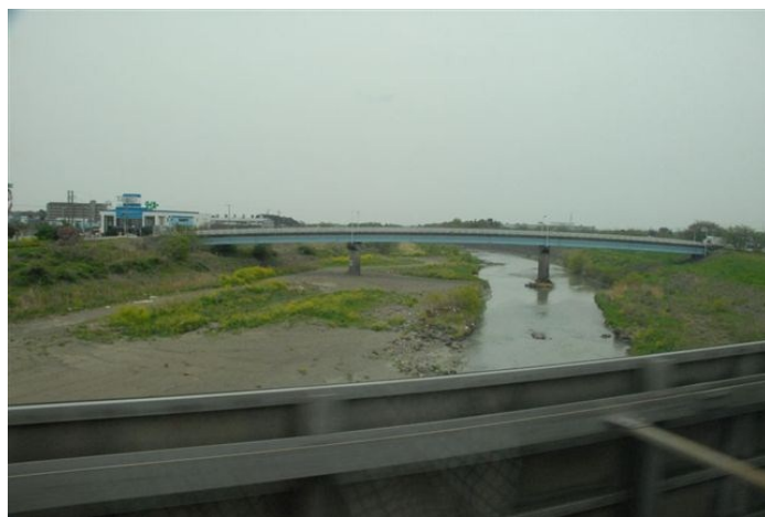
Photo 2. An example of setback dikes to contain a river channel constructed in Japan. This approach preserves fluvial processes and shoreline habitats while protecting upland agricultural and urban development (Photo credit Gary Williams).
